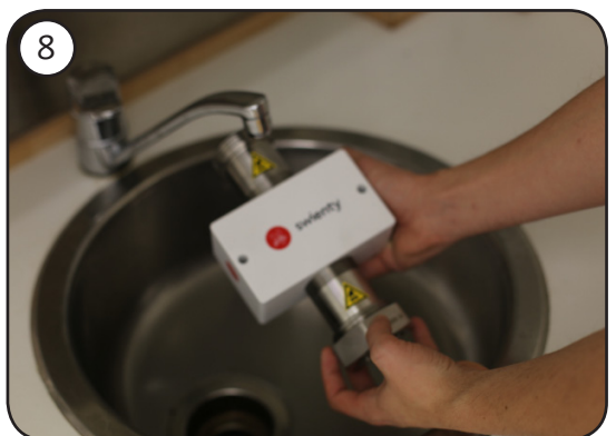
Remove the fitting below (Nut for BS fitting).
